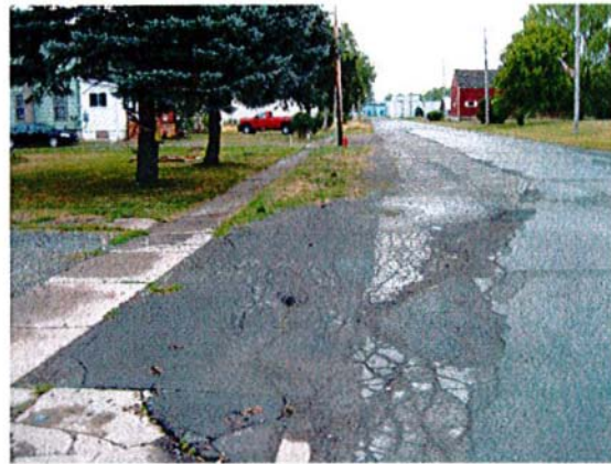
North side of Main Street near Pallister showing broken, uneven pavement sections, lack of curbing and insufficient drainage.
