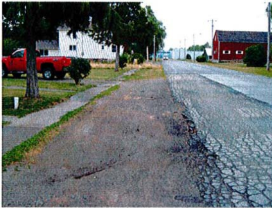
North side of Main Street near Pallister showing broken, uneven pavement sections, lack of curbing and insufficient drainage.
